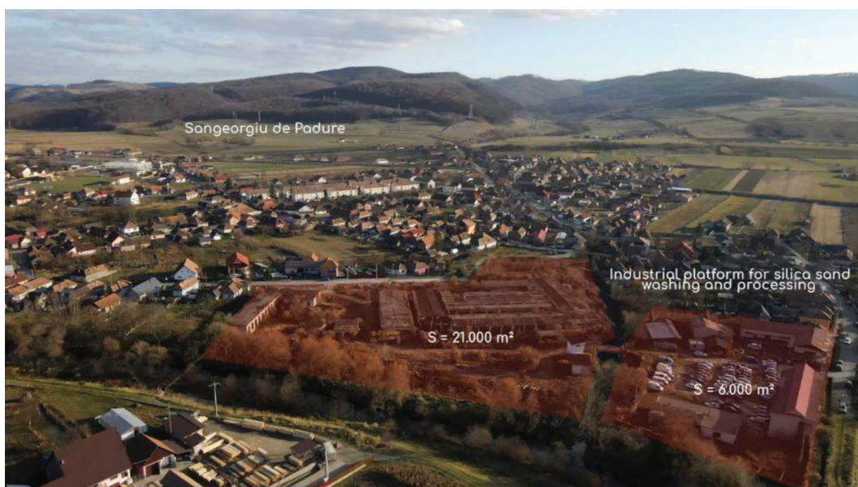
20. fig. – Sangeorgiu de Padure industrial platform
